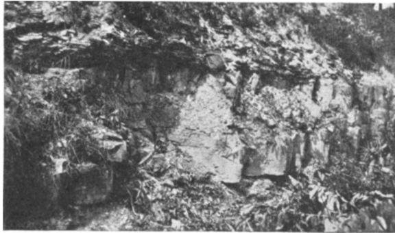
FIG. 4.—The Prout or Encrinal limestone overlain by the Huron shale at Slate Cut along the Lake Shore and Michigan Southern Railway three miles east of Sandusky, Ohio.
